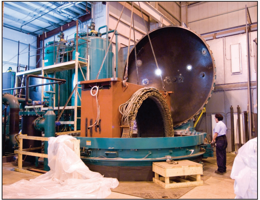
Repaired stator being lowered into HIEC VPI tank
