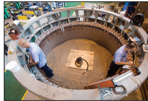
Connecting stator winding of a Hydroelectric Generator
